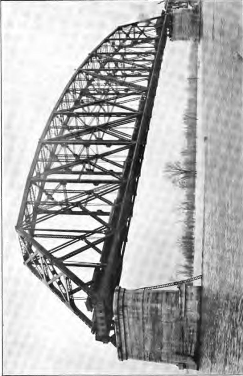
Fig. 150. The Longest Simple Truss Span in the World. Span 720 feet. C. B. & O. R. R. and N. C. & St. L. Ry. Bridge over the Ohio River at Metropolis, Ill. The Photograph was taken in 1917 especially for this illustration and before adjacent span on the left was erected.
